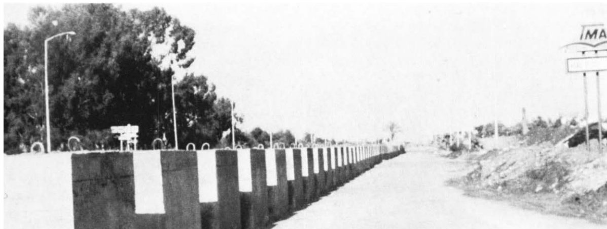
Shown in this photograph is one part of the Dragon's Teeth perimeter surrounding the 22d MAU's positions at Beirut International Airport. Nearly 800 were emplaced.
