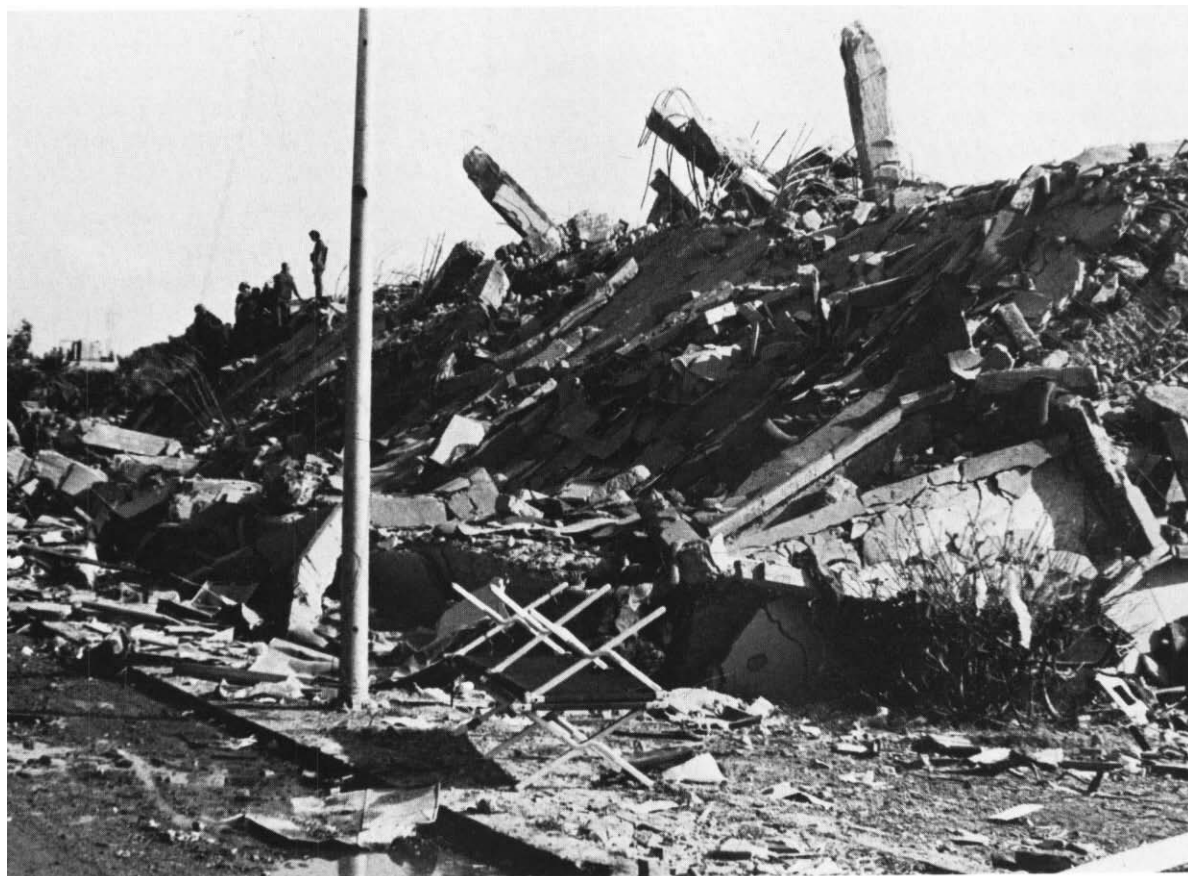
Some views of the destruction following the bombing of the BLT headquarters building.
